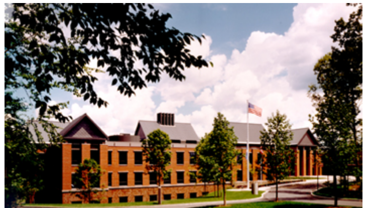
The Duracell Headquarters on Research Drive in Berkshire Corporate Park.
