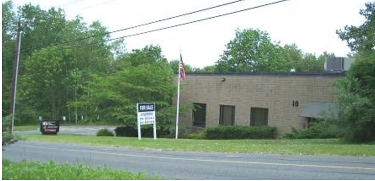
16 Commerce Road, one of the GE buildings on the market
